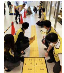
Employees laying tactile paving
